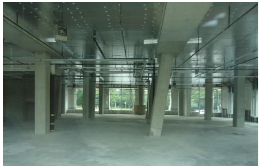
Figure 7: Sloped Columns in Retail Space
